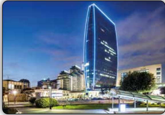
PORT BAKU TOWERS
