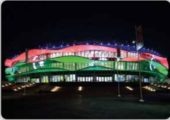
NATIONAL GYMNASIUM ARENA, BAKU
