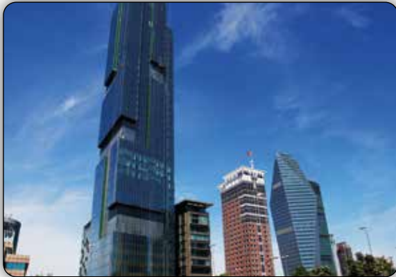
LEVENT 199 TOWER, ISTANBUL
