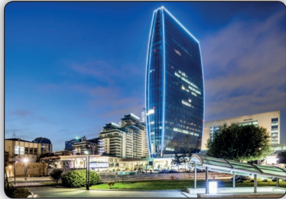
PORT BAKU TOWERS
