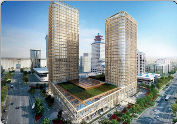
TALAN TOWERS, ASTANA
