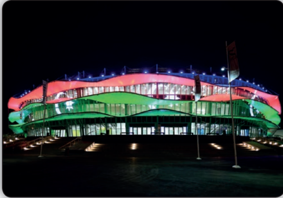
NATIONAL GYMNASIUM ARENA, BAKU
